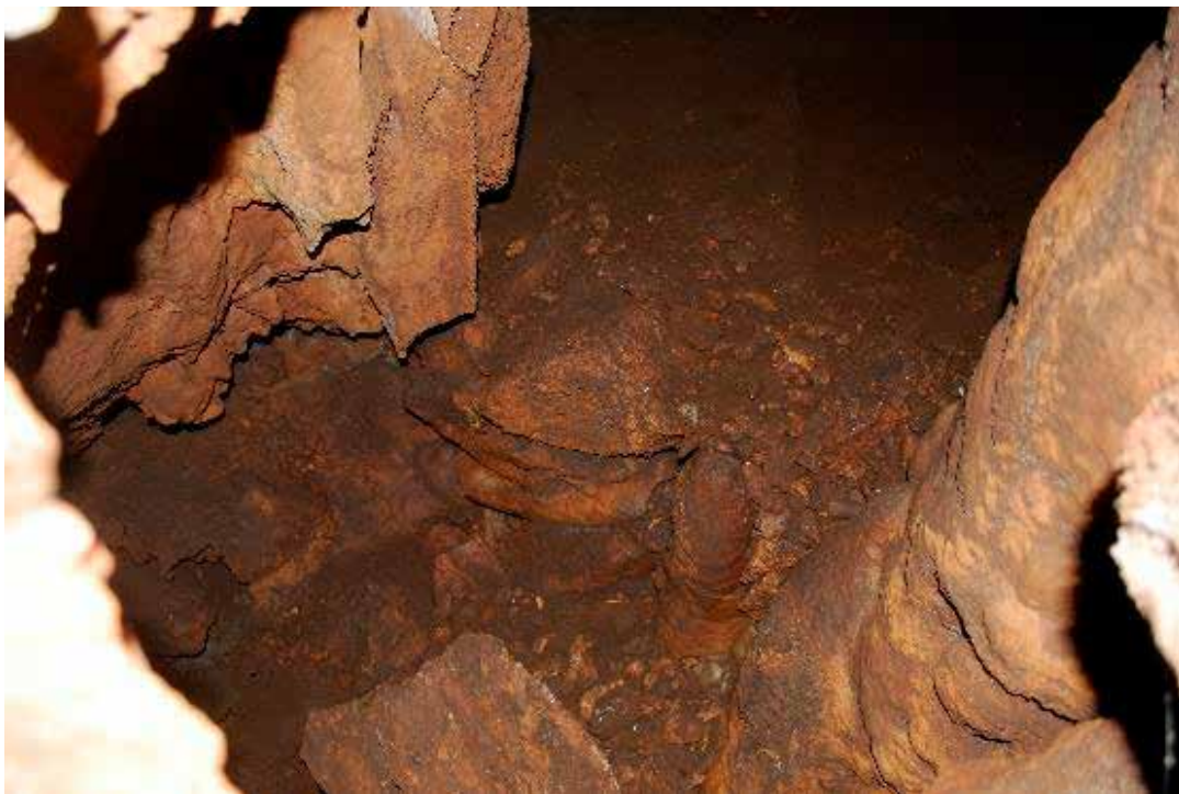
Figure 14: A built wall supporting the platform of area CC (the dark area at the top right)
